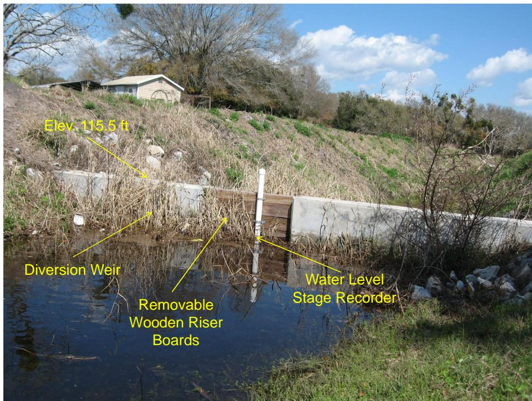
Figure 1-5. Diversion Weir Structure in the Northwest Ditch.
