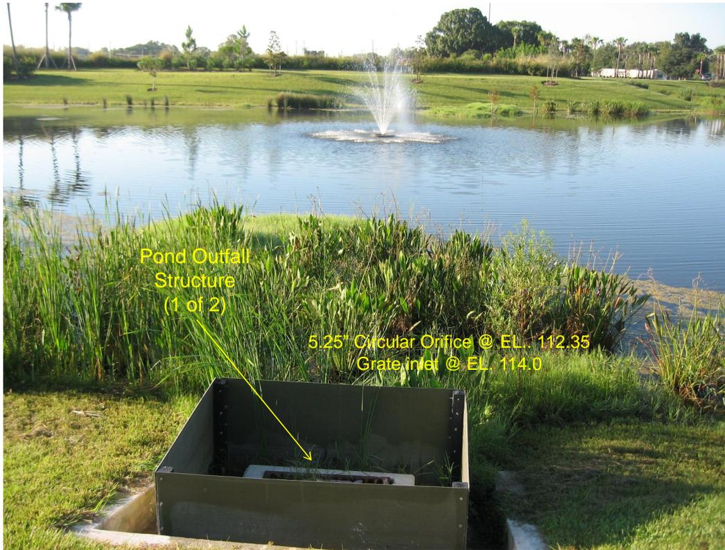
Figure 1-8. Outfall Structure for the Pioneer Key Pond.
