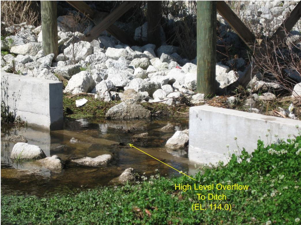
Figure 1-9. High Level Overflow Structure on the Northeast Corner of the Pioneer Key Pond.
