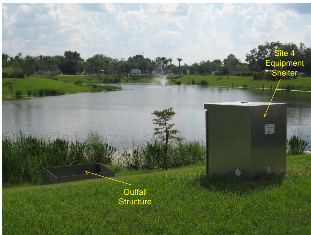
Figure 2-6. Monitoring Equipment Installed at the Pond Outfall (Site 4).
